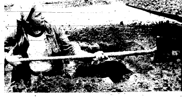
MARLENE VENTEICHER digs her work as the first female member of the City of Wayne street department, although she will leave the department to become a freshman at Wayne State College this week. She joined the department in May. Here she is helping to repair a troublesome storm sewer.
